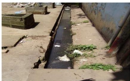
**Fig. 5:** Blocked drainage channel
