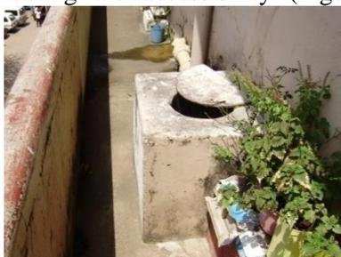
**Fig. 2:** Insufficient accessibility due to the refuse chute
